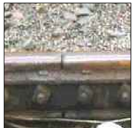
This joint has been shimmed. Look for the small tabs just above the fishbolts.
