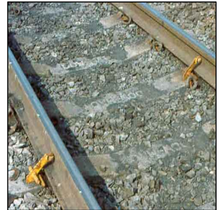
CWR on rollers and supported with sidearms
