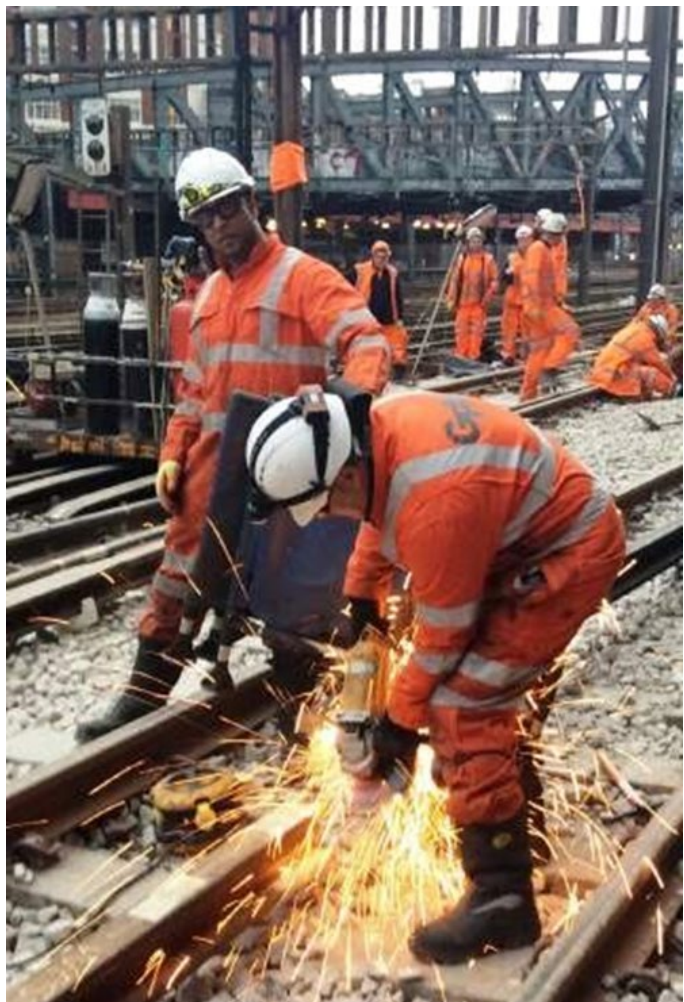
Example of hot working
