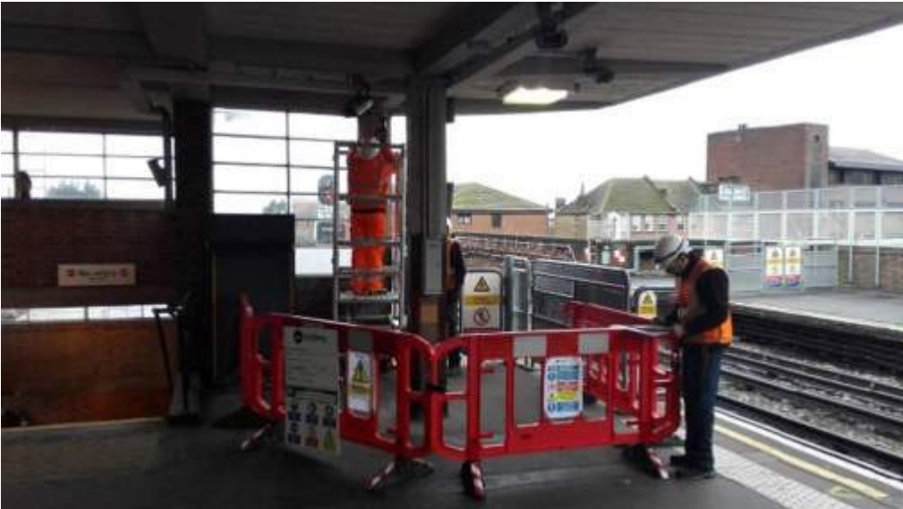
Example of a worksite on a station platform
