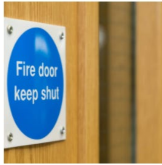
Fire door - must keep shut
