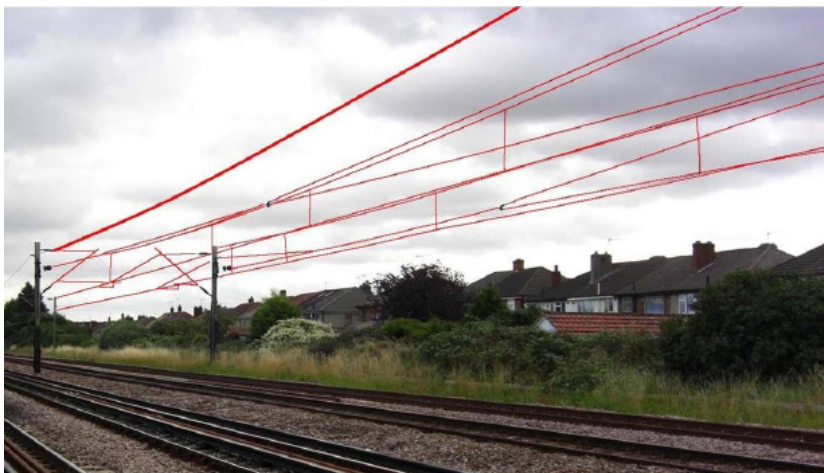
Example of Overhead Line Equipment
