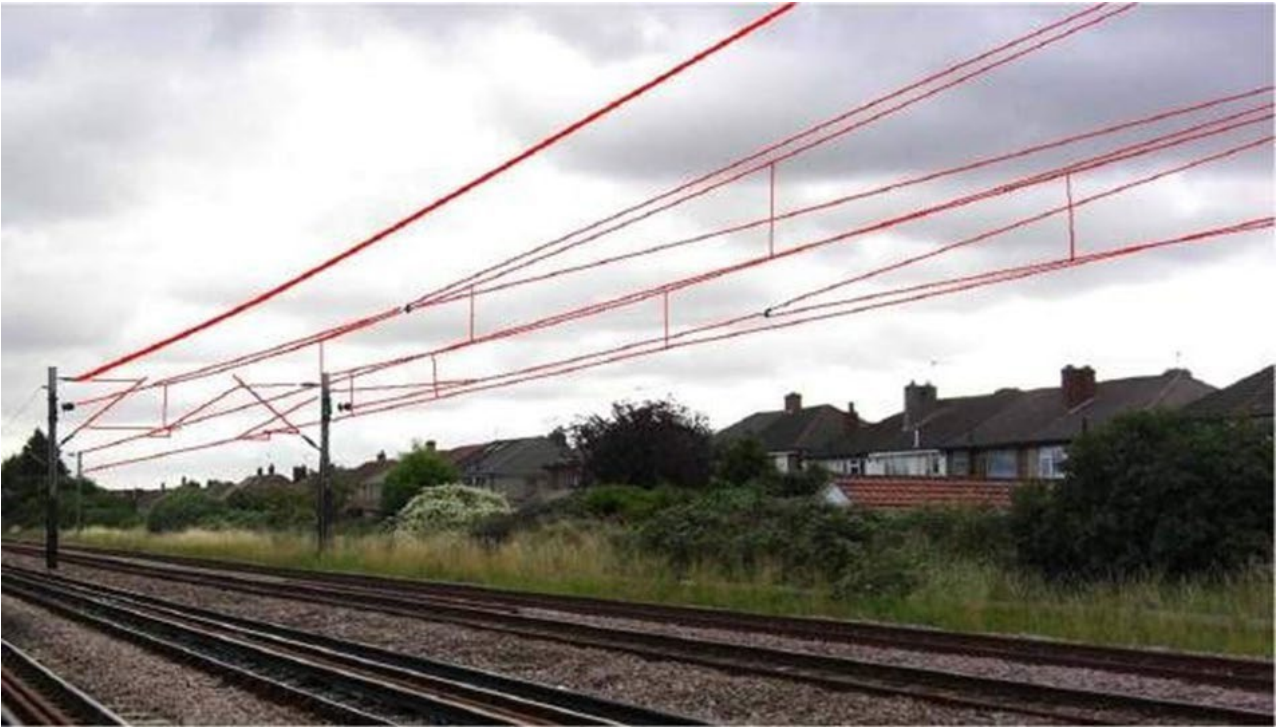
Example of Overhead Line Equipment
