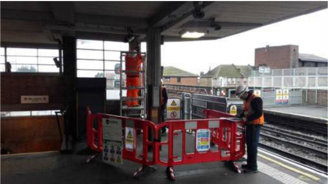
Example of a worksite on a station platform
